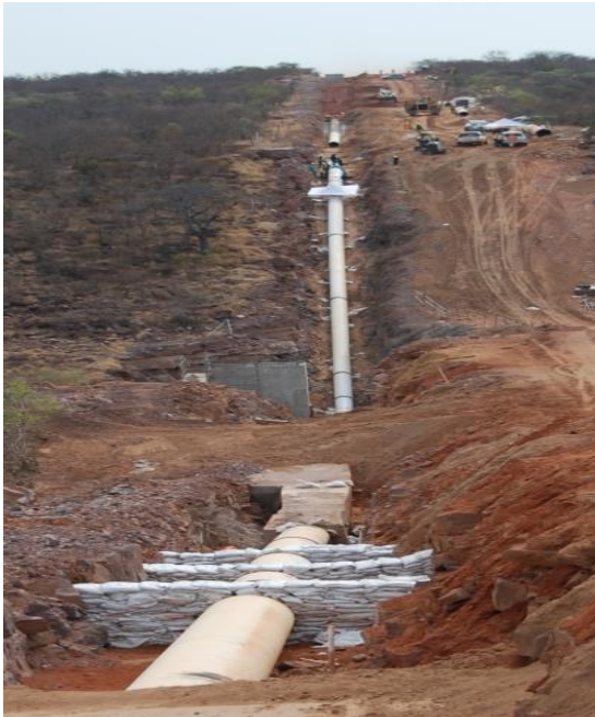
Rising Main Pipe Laying
