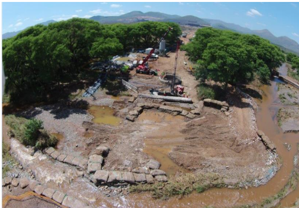
Steelpoort River Crossing
