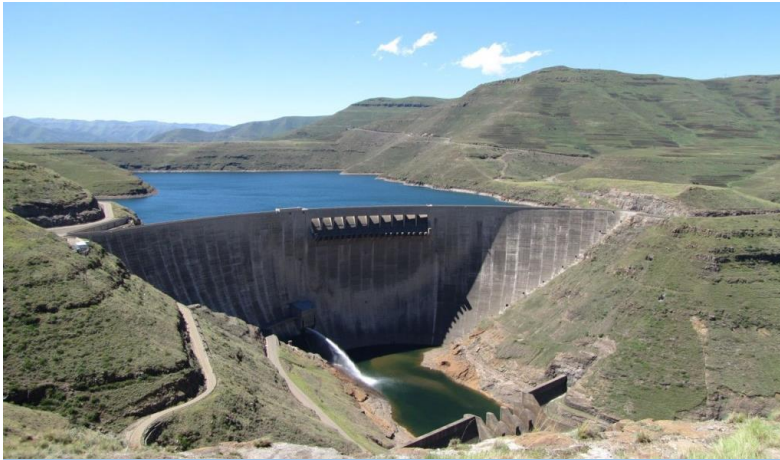
Phase 1A (completed 1998): Katse Dam
