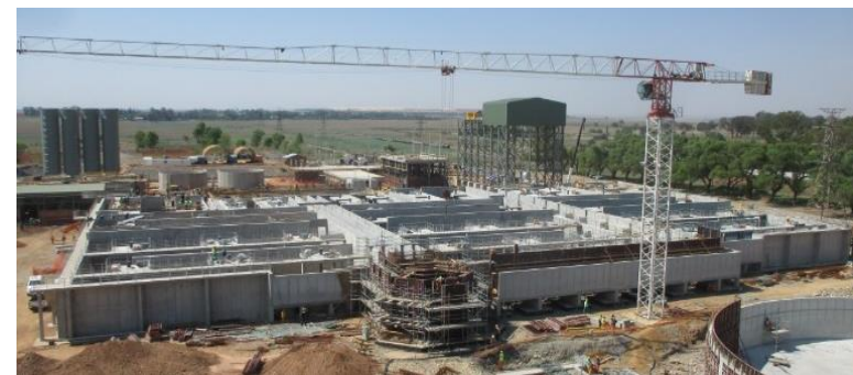
Eastern Basin: Reactors under Construction
