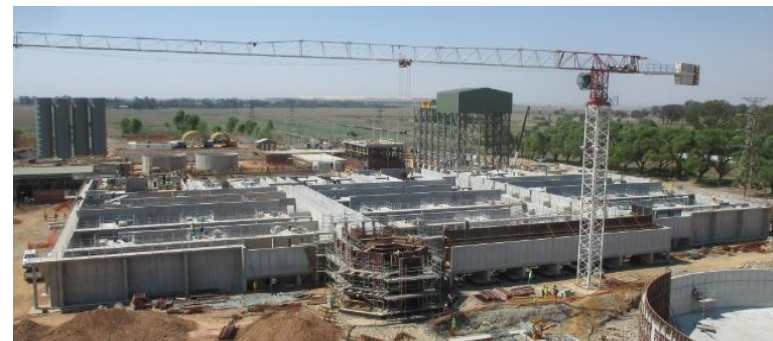
Eastern Basin: Reactors under Construction
