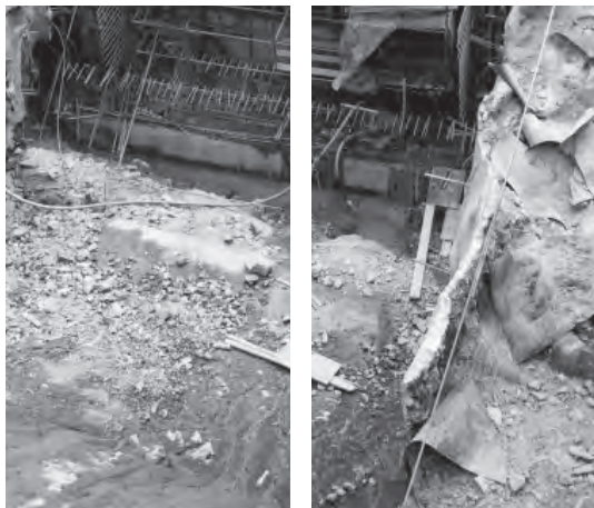
Permanent abstraction works: VRESAP
