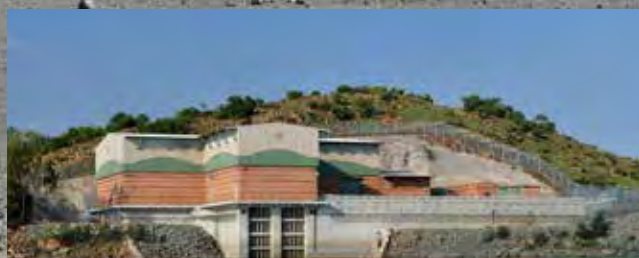
VRESAP intake at Vaal Dam
