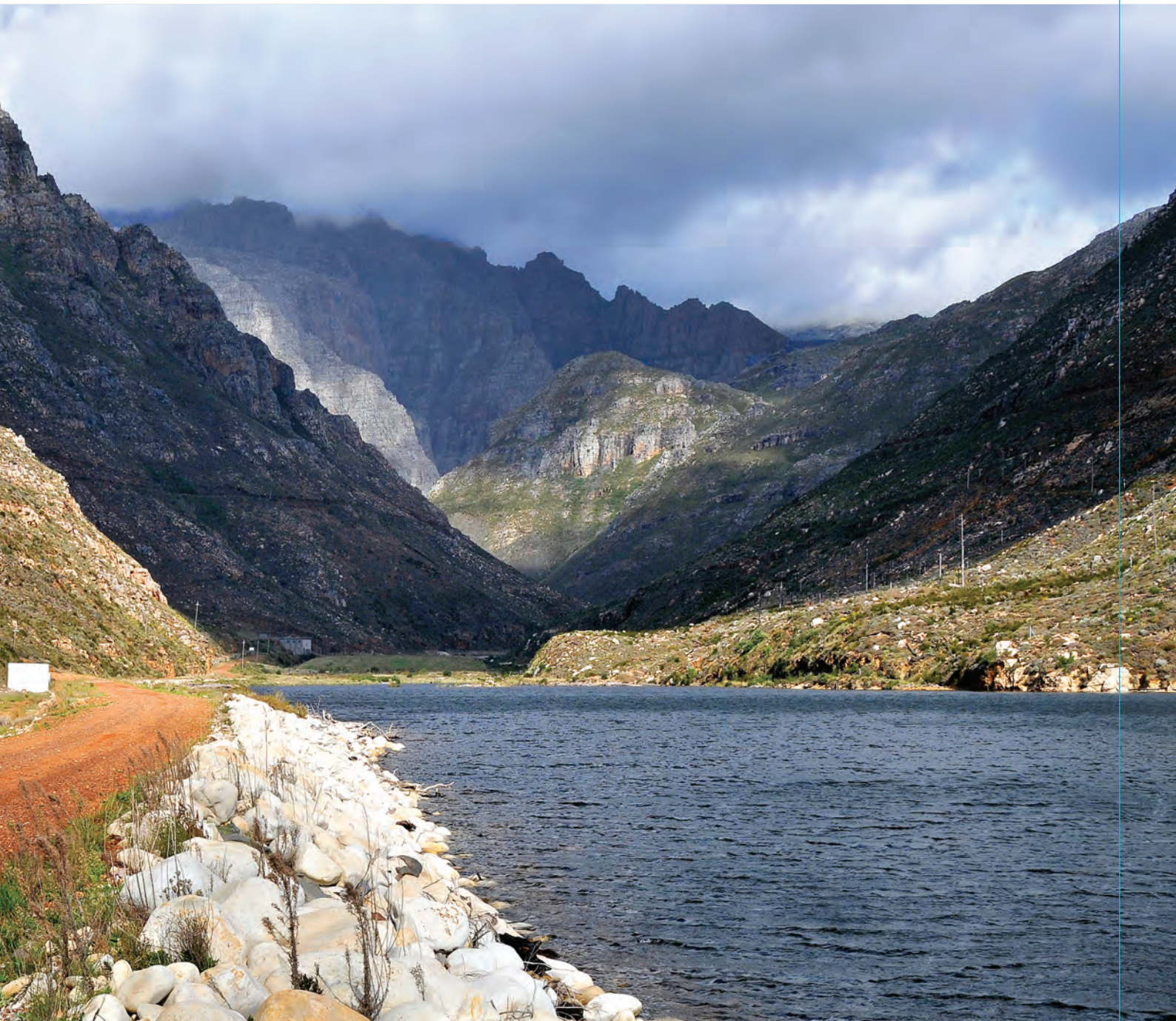
Berg Water Project: Views of the dam from Robertsvlei
