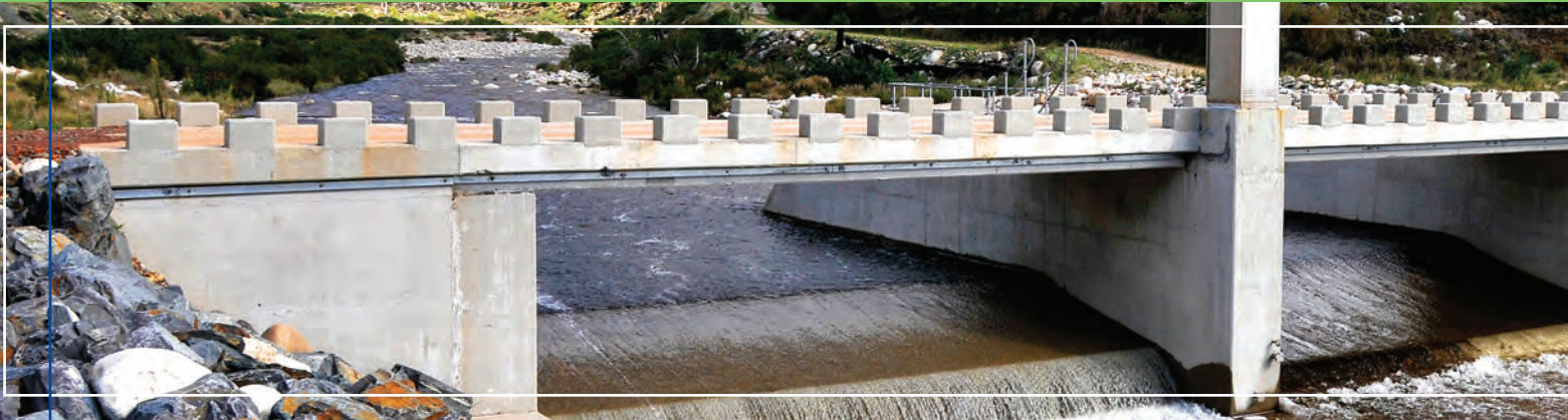
Berg Water Project: Upstream weir at Assegaaibos
