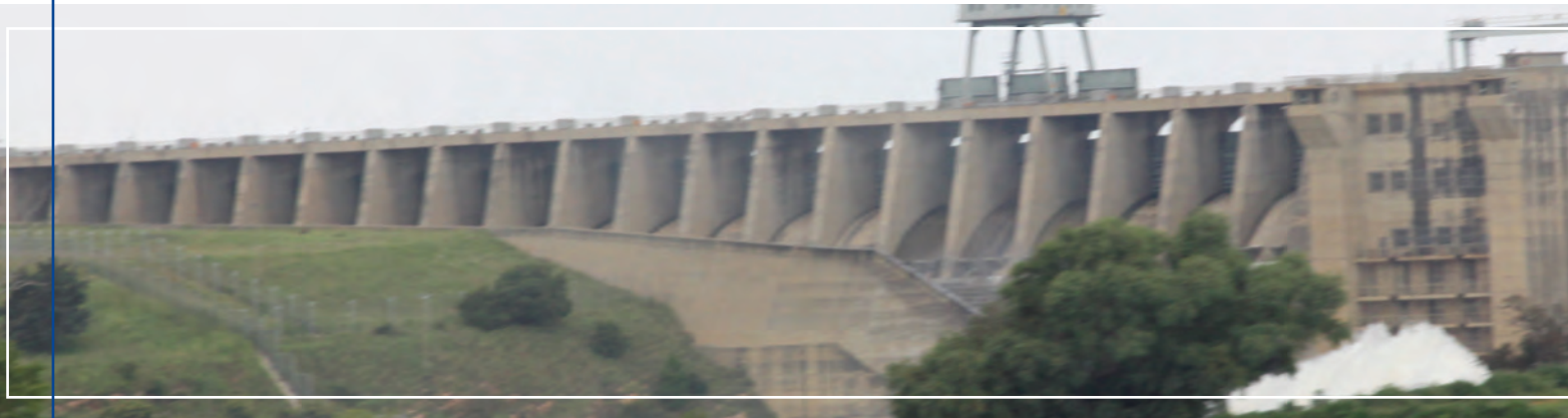
The Vaal Dam: The Vaal River Eastern Subsystem Augmentation Project pipeline transfers water from the Vaal Dam to the diversion structure at Knoppiesfontein
