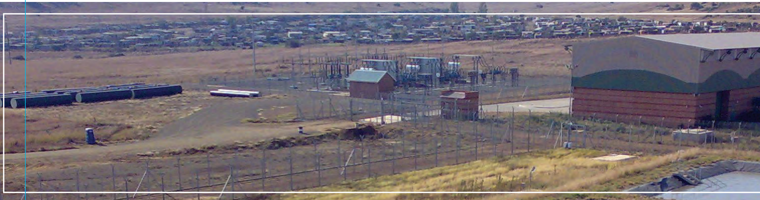
Project pump station showing Mamello Township (one of the beneficiary communities) in the background
