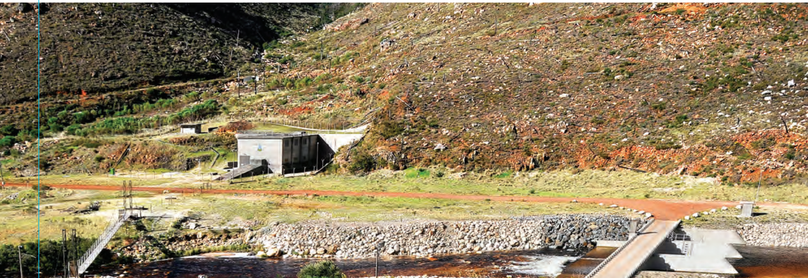
Berg Water Project: Views of the dam from Robertsvlei
