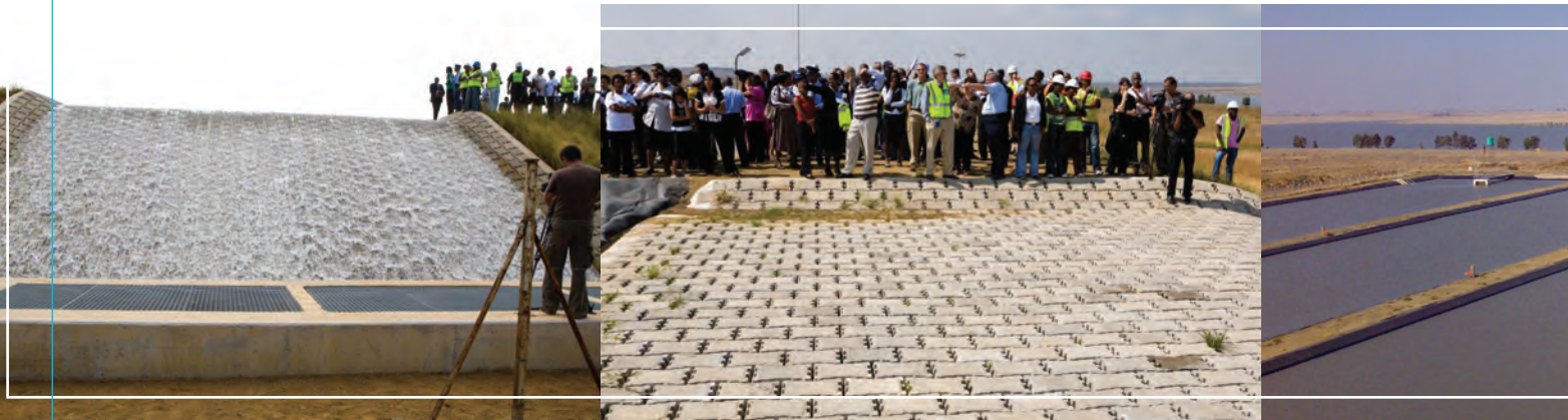
Vaal River Eastern Subsystem Augmentation Project: Stakeholders witnessing a spillover demonstration from the balancing dams during the Water Delivery Celebration in April 2009
