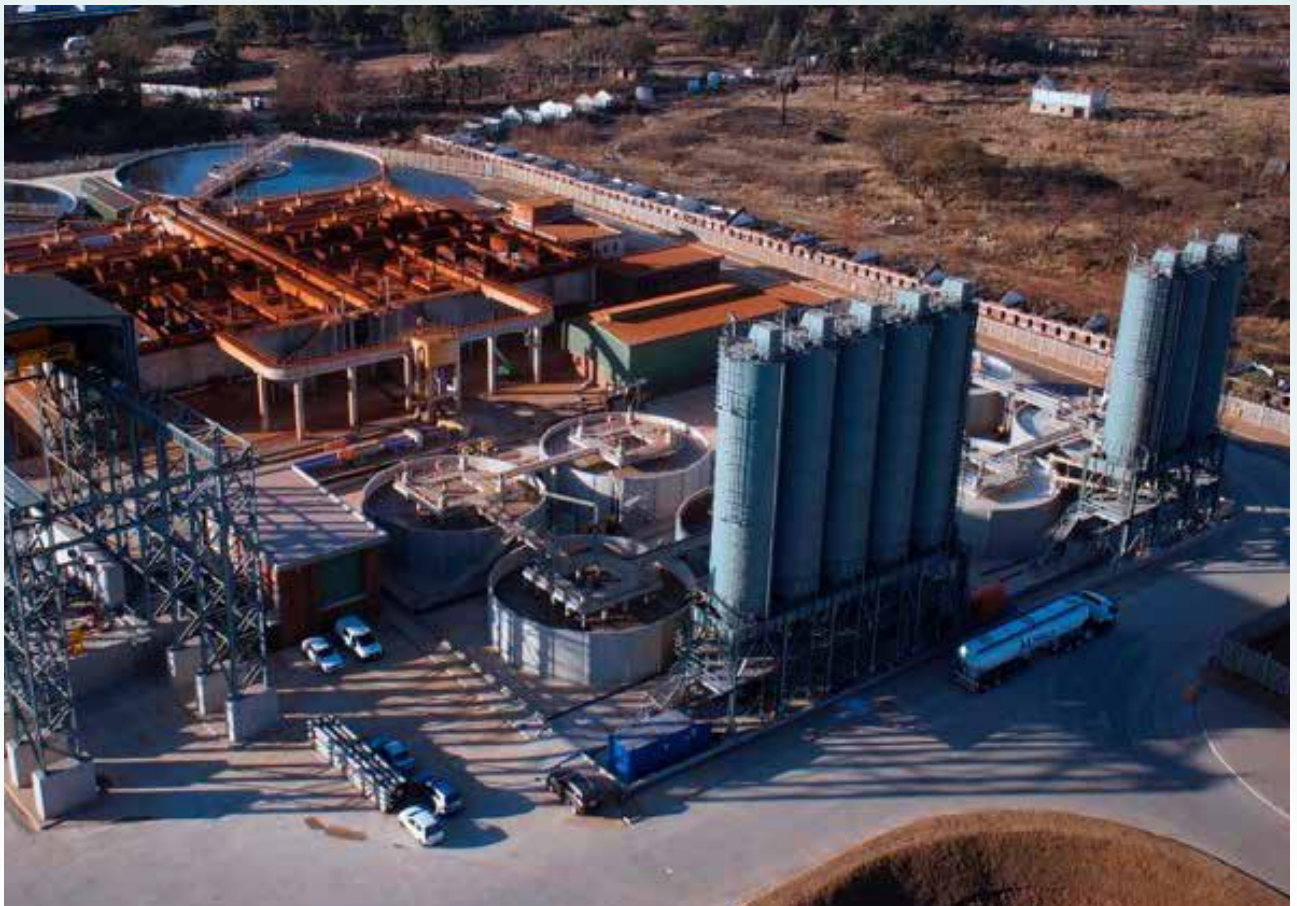
AMD: Central Basin high density treatment plant
