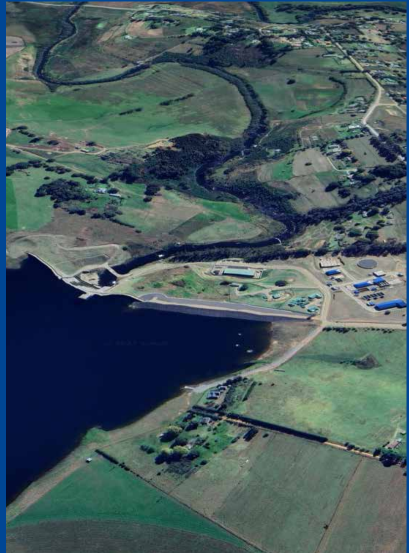
Spring Grove Dam and Rosetta Water Treatment Works
