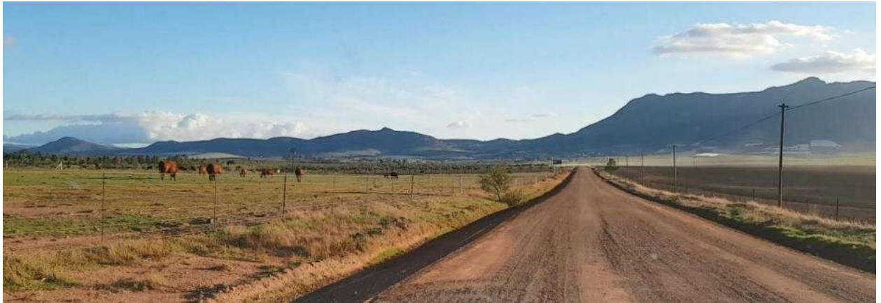
Gravel Road in very good condition
