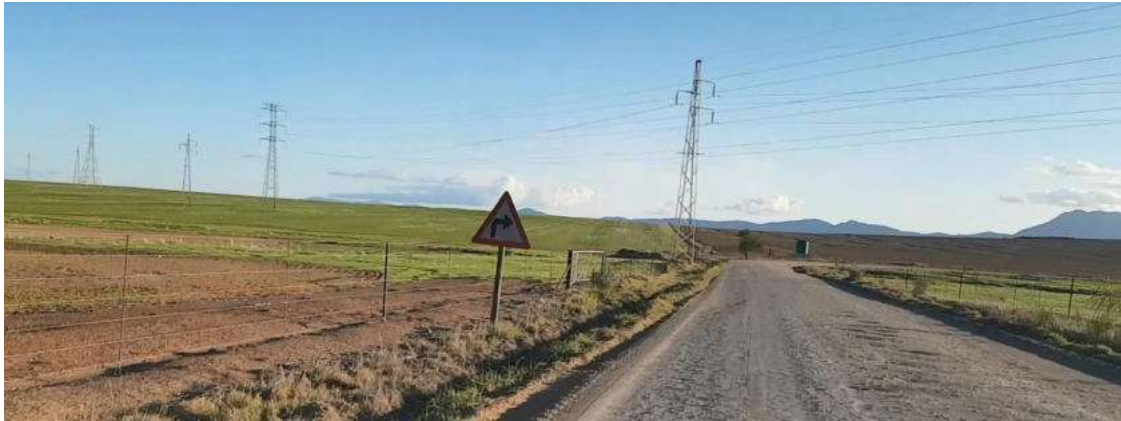
Gravel Road in very poor condition
