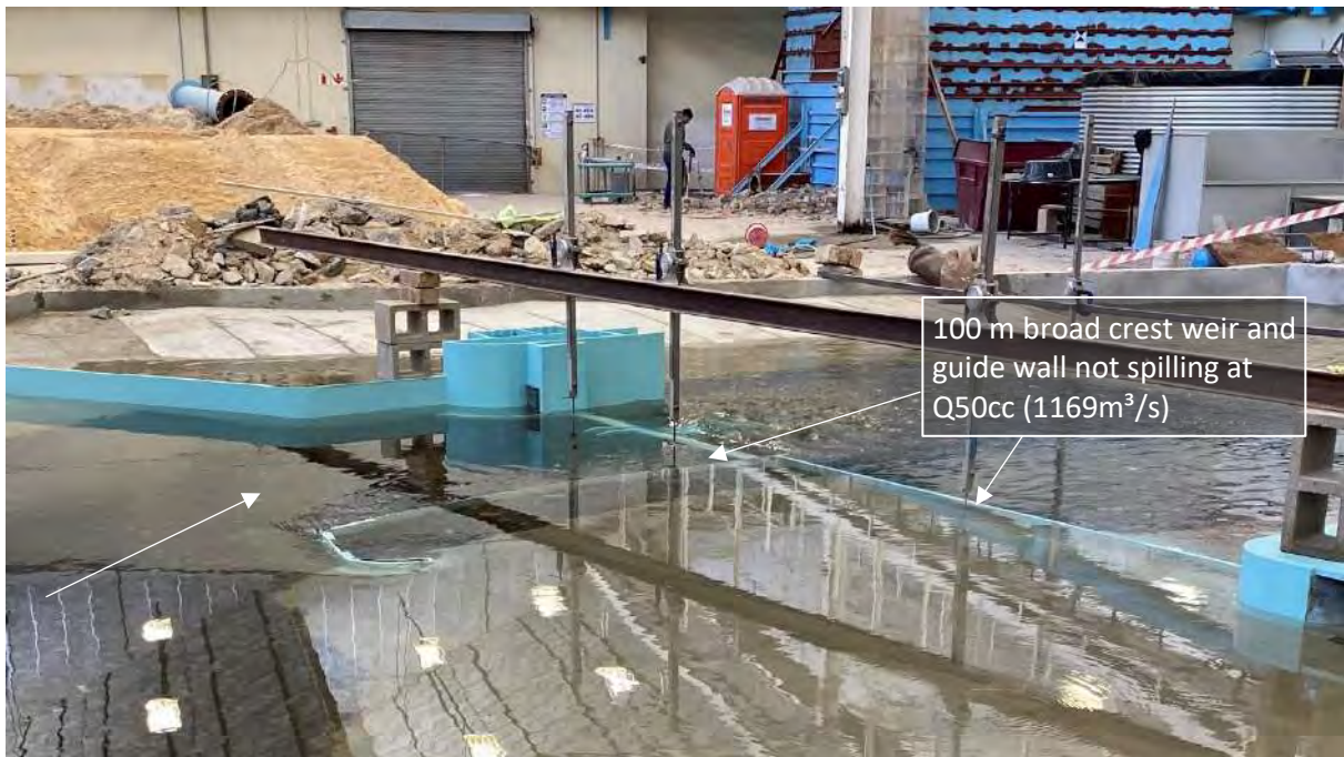
Figure 9-19: Q50cc (1169 m 3 /s) guide wall diverts flow towards the 60 m weir and abstraction works
