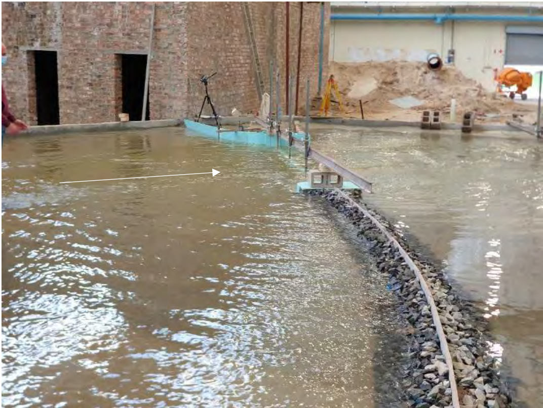
Figure 9-7: Weir with 4 notches, abstraction works and berm during the RMF (4 494 m 3 /s) as viewed from the right bank side
