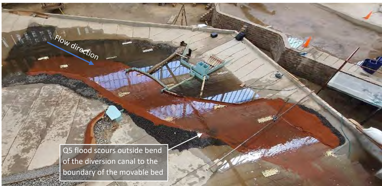
Figure 10-21: Modified option C layout of the diversion canal during the Q5 flood
