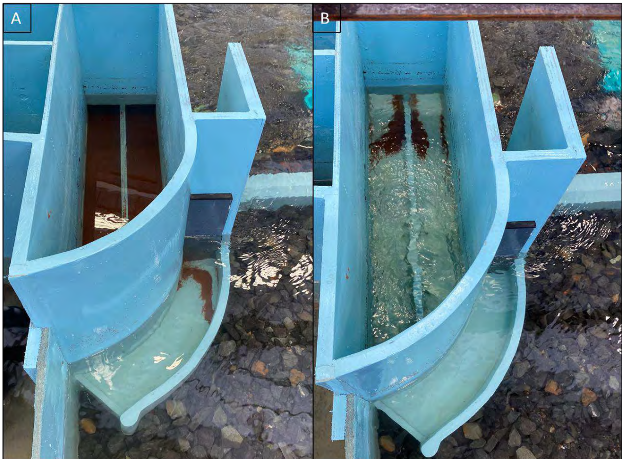
Figure 9-23: Gravel traps are flushed at Q10cc (613 m 3 /s). Figure A shows gravel traps before flushing and Figure B shows gravel trap during flushing with both sluice gates open
