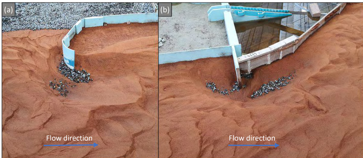
Figure 10-23: Scour around the right bank guide wall, a) upstream and b) downstream, after the Q5 flood
