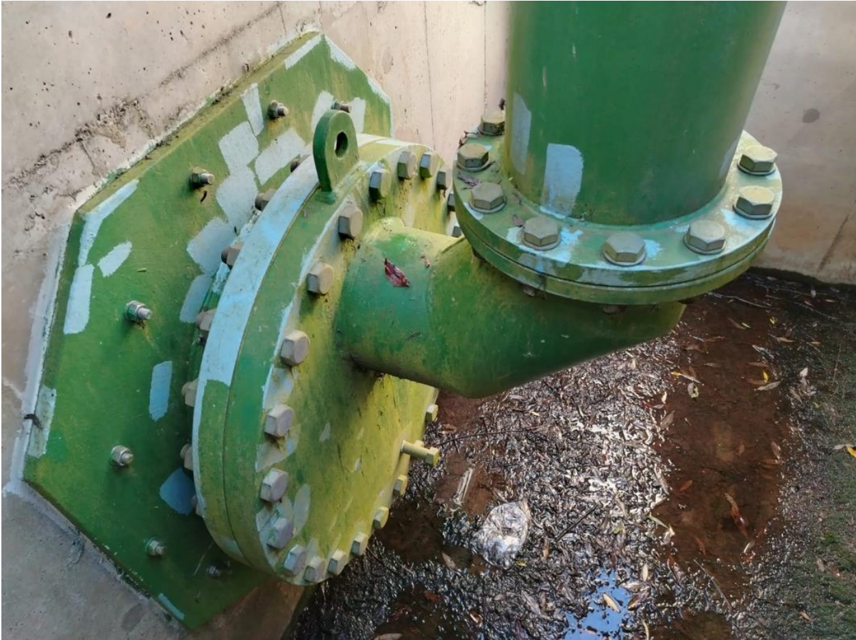
Dihlabeng municipal water connection to be removed and reinstated Picture No 06
